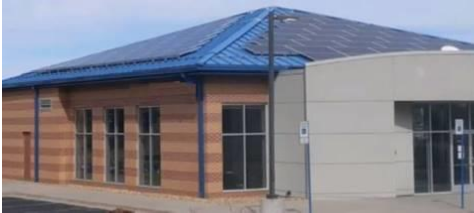
Sample photo of a completed JP Morgan Chase solar project
