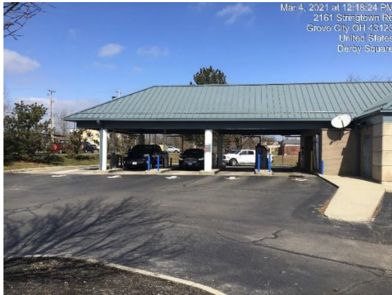
View from the Southeast corner of the parking lot looking North
