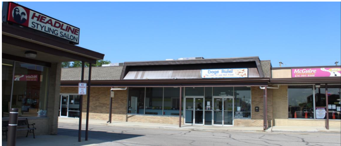
Existing Building Front and Rear Fenced Area
