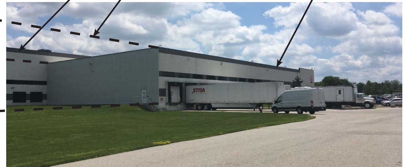
AREA OF ADDITION LOOKING SOUTHWEST
