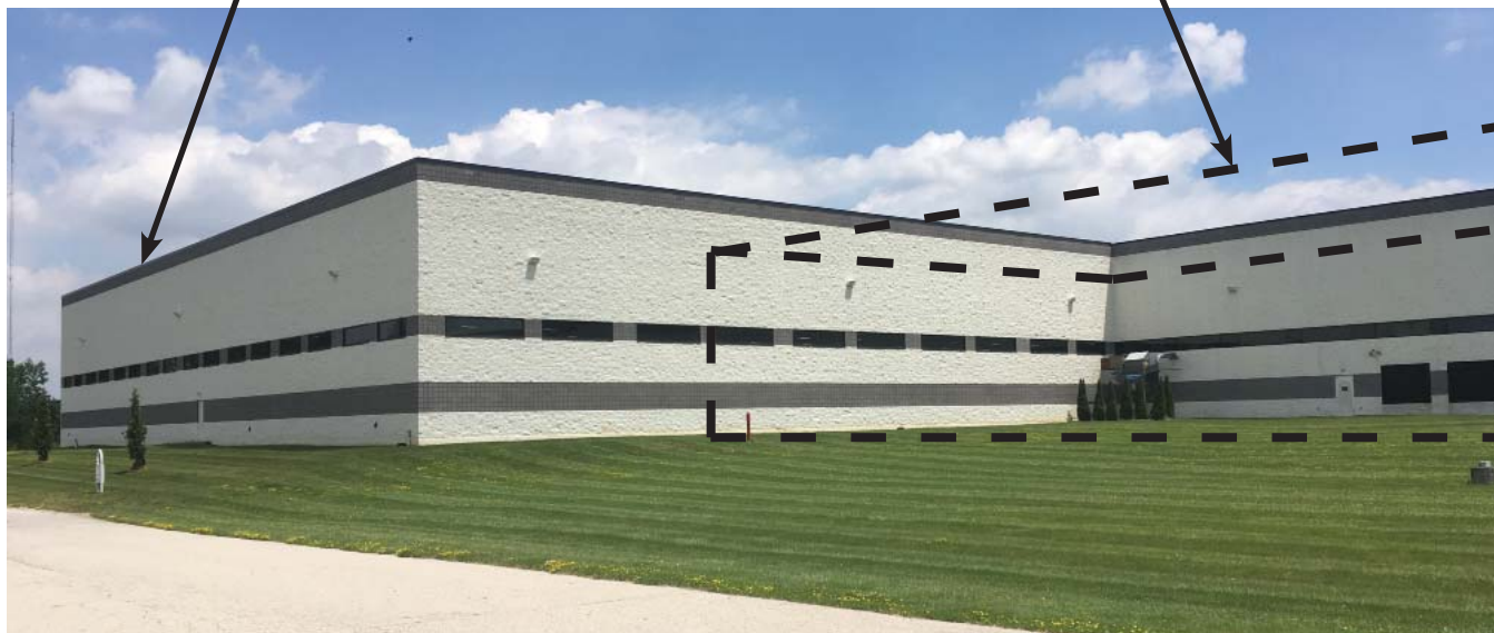
AREA OF ADDITION LOOKING SOUTHEAST
